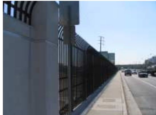
Crash rated stucco covered CMU block wall.
