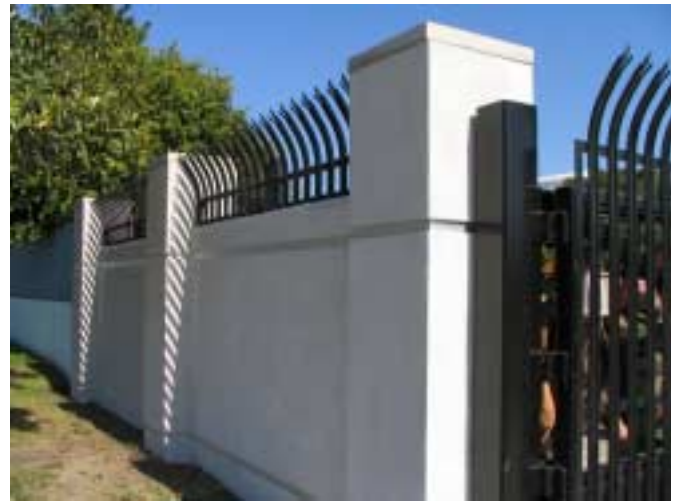
Crash rated stucco covered CMU block wall.
